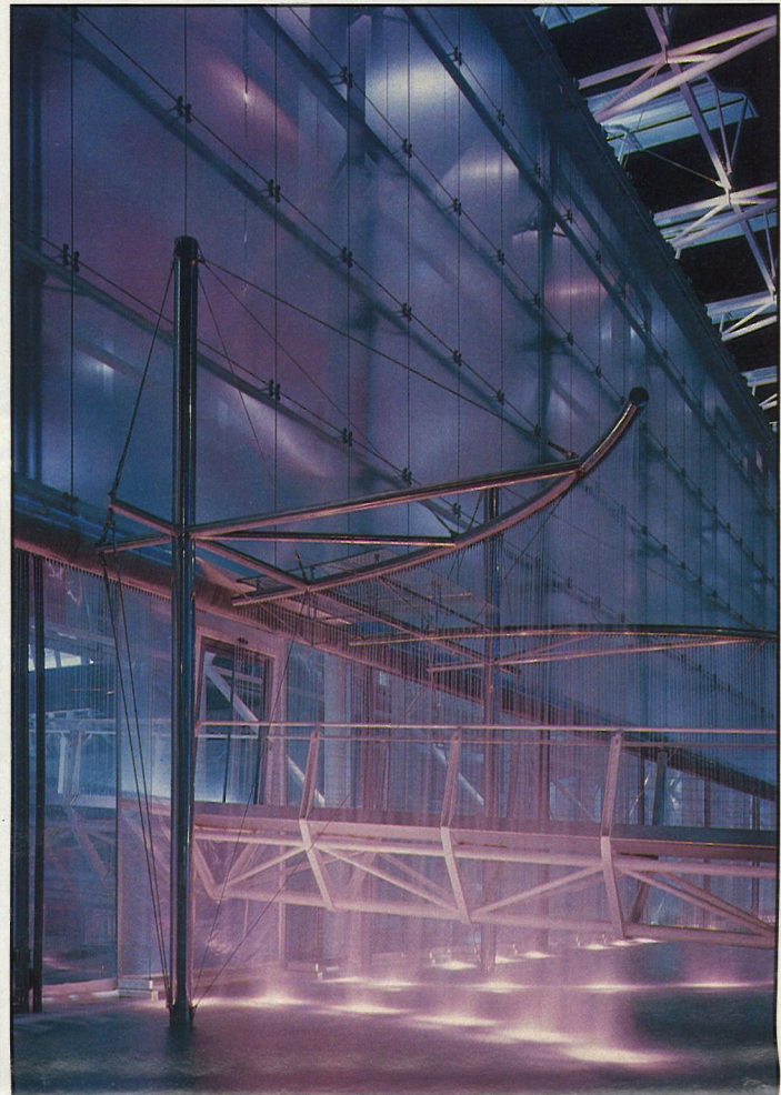
The entrance area with its 3kW tungsten underwater fittings.
